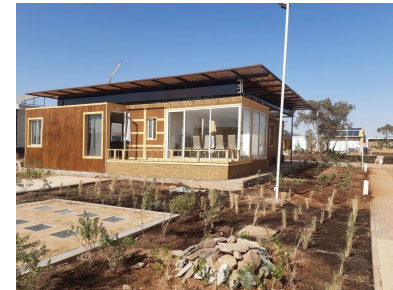
Jua Jamii (Tanzania): Energy Efficient Affordable Homes
